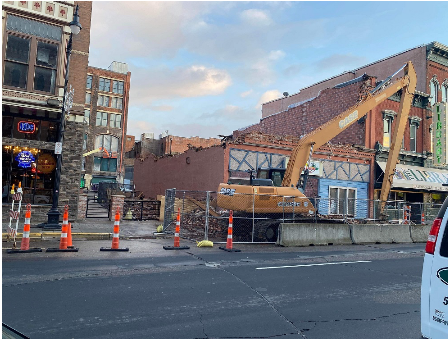
Jehlen Building demolition. Photo courtesy of Laura Godden.
